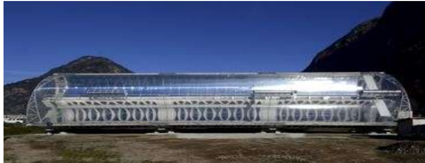
Figure 18. Multi-Junction Solar Array Enclosure.
